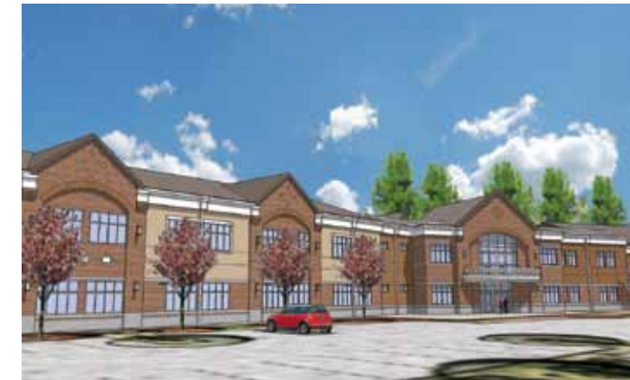
Entrance to the new Upper School
