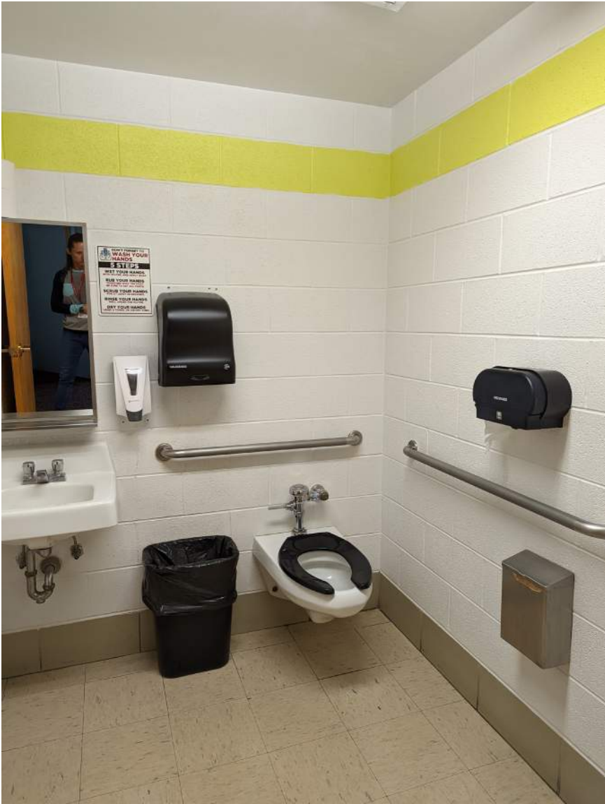
EXISTING STAFF TOILET
