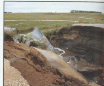
Culvert wash-out on the Ward road
