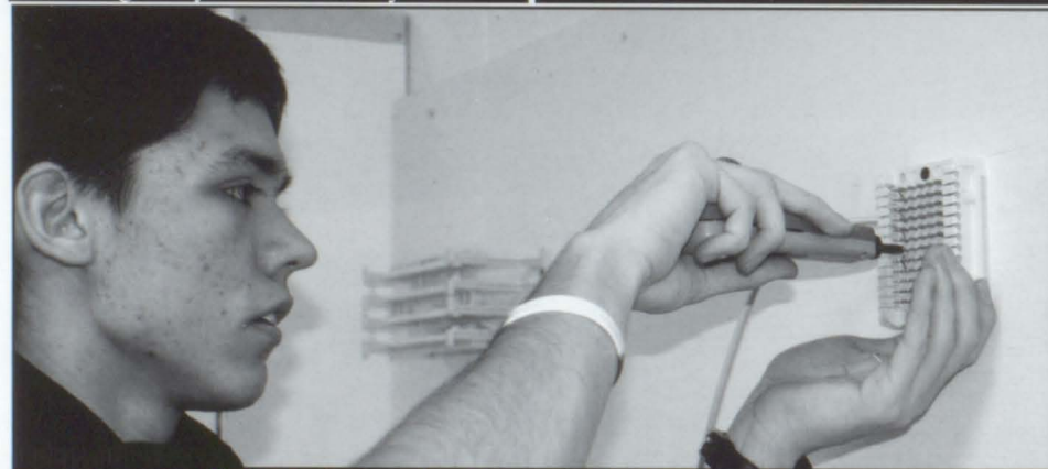
Skyler Earley punches down a 66-block in C-Tech class.
