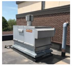
All existing packaged rooftop units installed through the 2015 and 2019 equipment upgrade projects utilize refrigerant type: R-410A. These units are in good operating condition.
