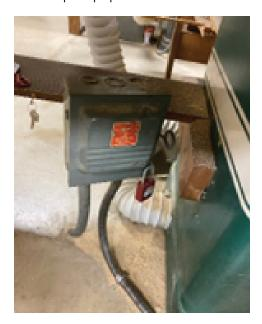
We did not verify if circuits contained independent grounding conductors. This should be done by a qualified electrical contractor or at a minimum verify grounding continuity in all circuits. It was common in schools in Wisconsin to use the conduit as a grounding system on some older facilities. Over time the conduit may have disconnected causing ungrounded circuit conditions. We always recommend a
