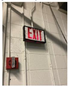
Ensure full egress lighting compliance throughout the facility and add light fixtures to the life-safety emergency panelboard as necessary.
