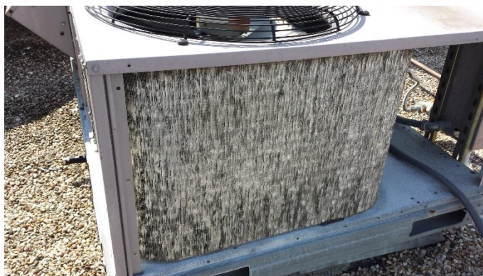
Figure 50. Damaged heat-exchanging fins on unit at Cedar Creek Elementary School.
