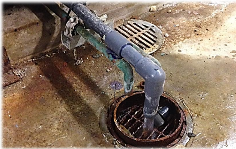
Figure 30. Typical cooling tower system blowing down.
