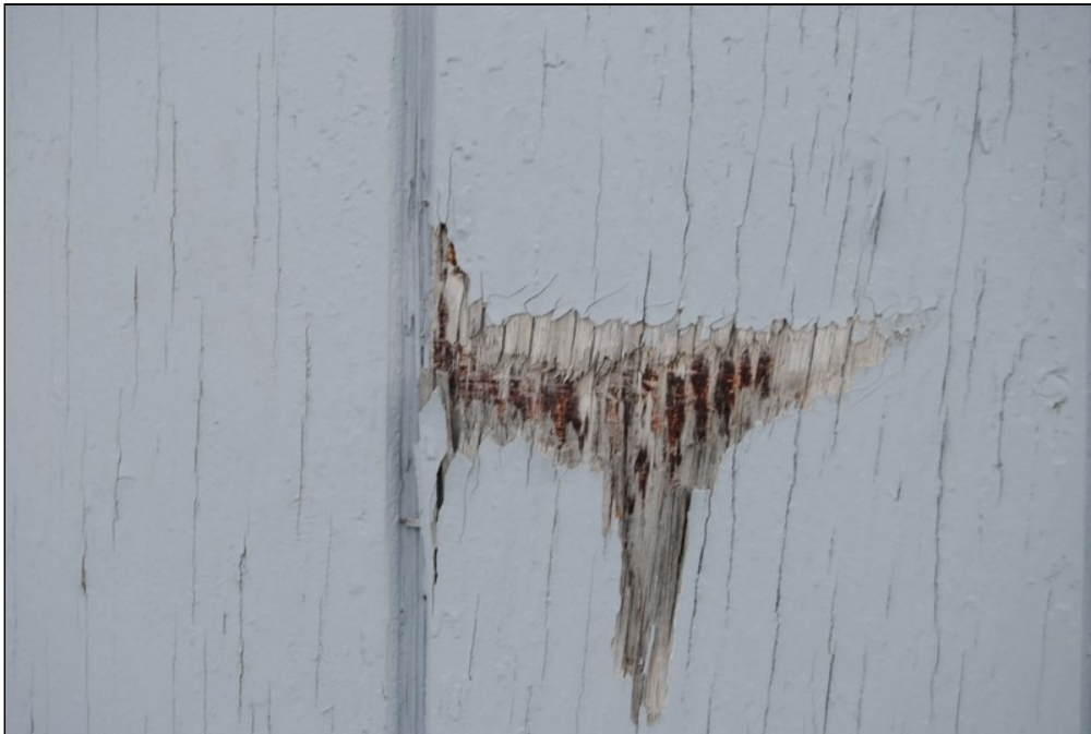
2 - deteriorating siding
