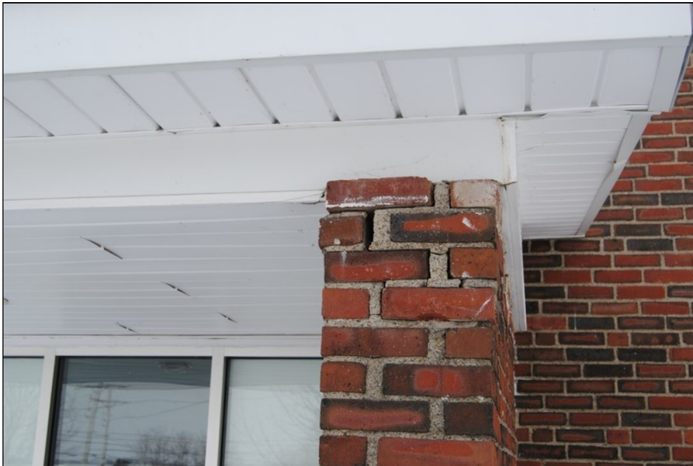
68 - deteriorated brick on pilaster
