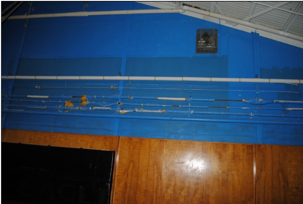
54 - damaged pipe insulation
