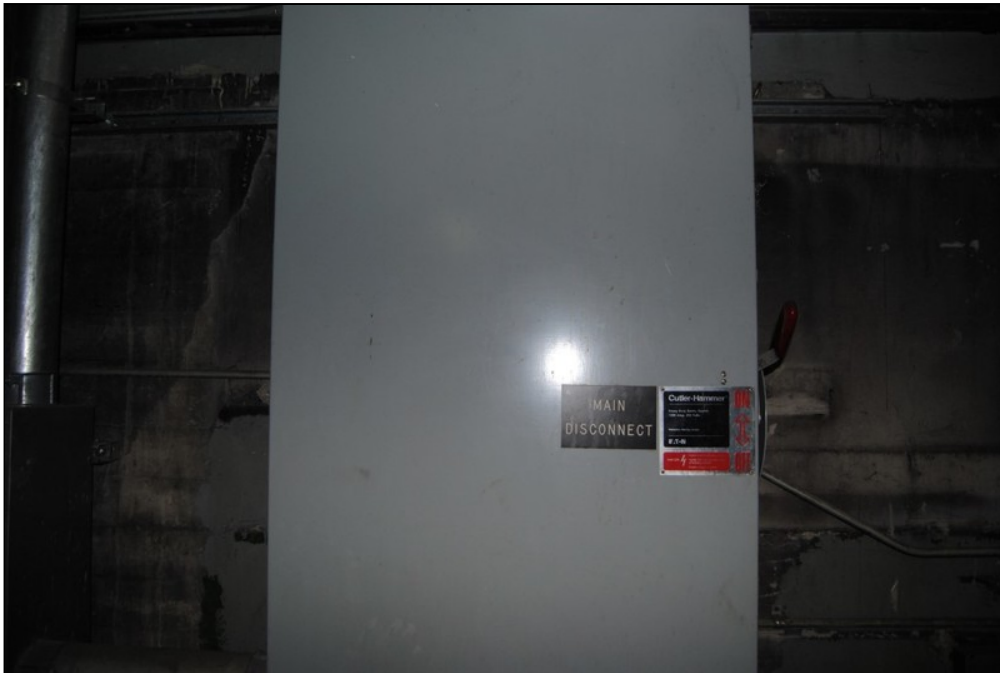
20 - main switch gear
