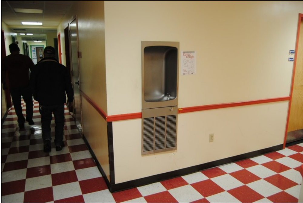
45 - non-ADA water fountain
