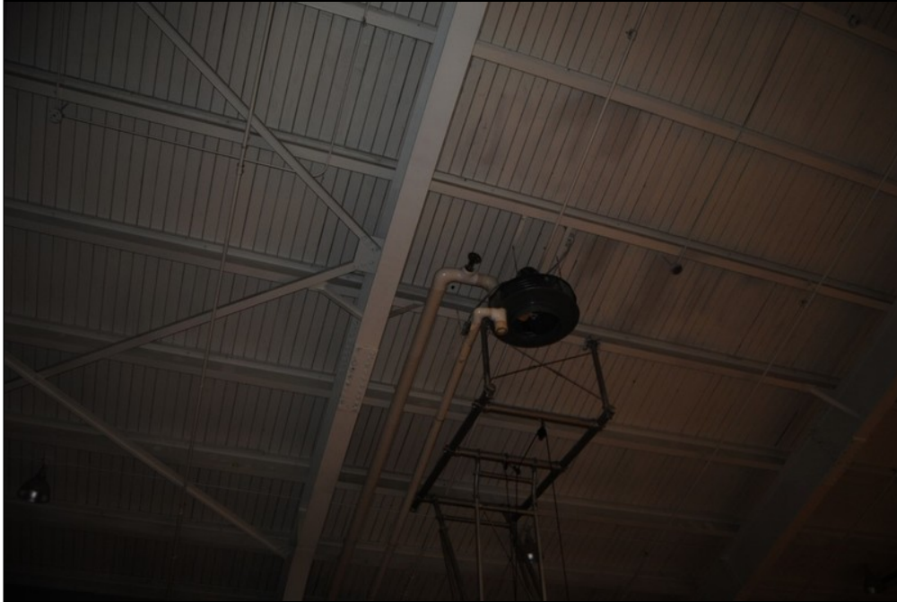
55 - ceiling space heater
