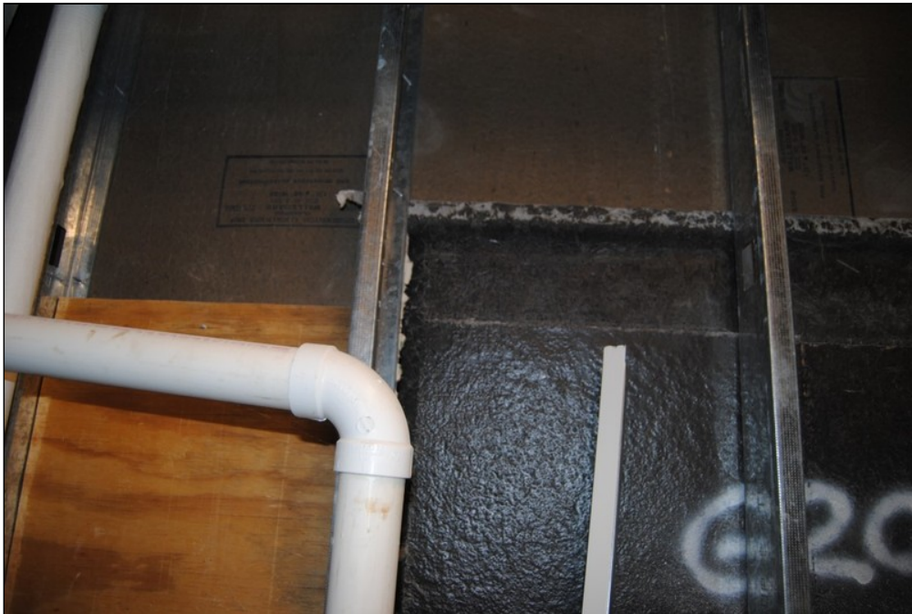
52 - interior wall framing
