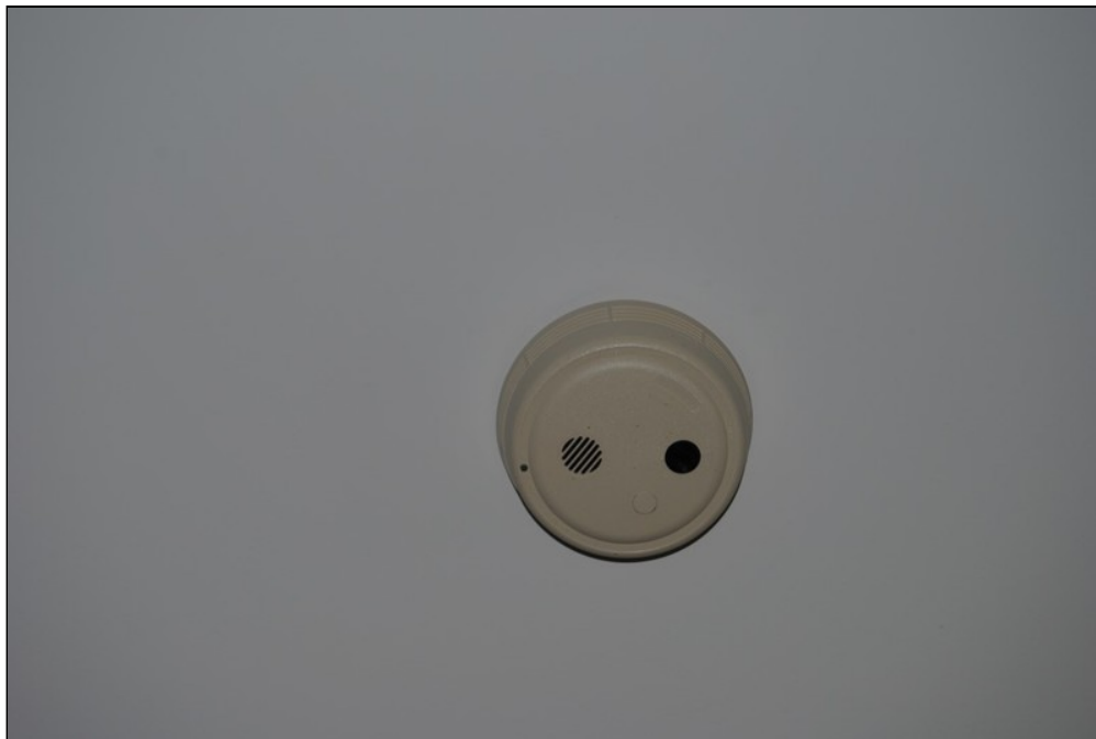
36 - room smoke detector
