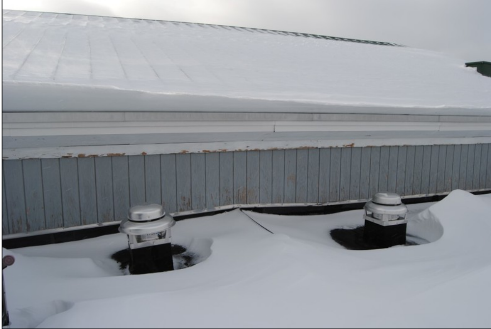
61 - roof top vents
