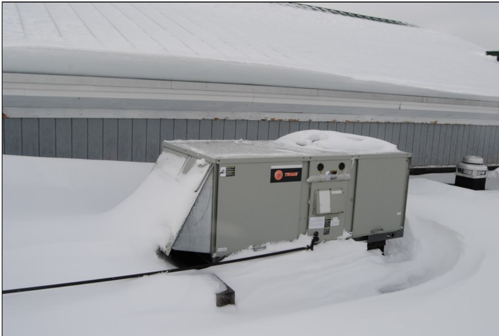
60 - roof top unit
