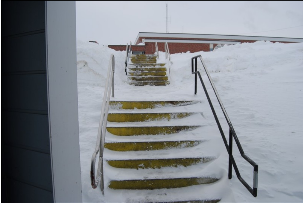
9 - south entrance stairs
