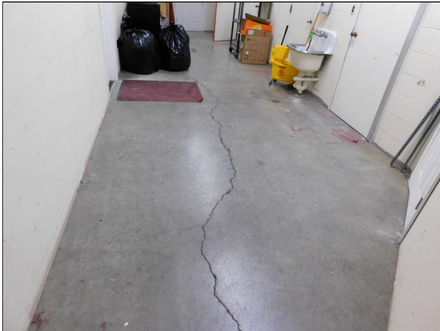
76 - cracked slab
