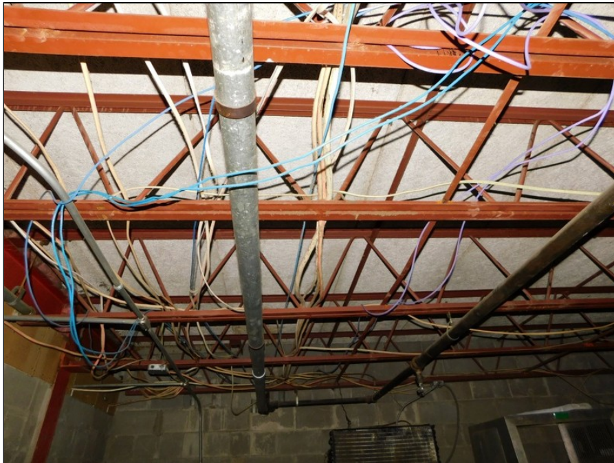
70 - Steel joist
