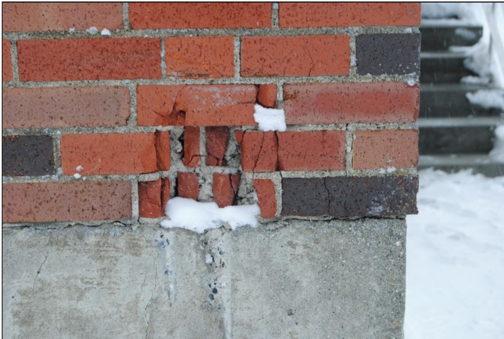
18 - damaged brick
