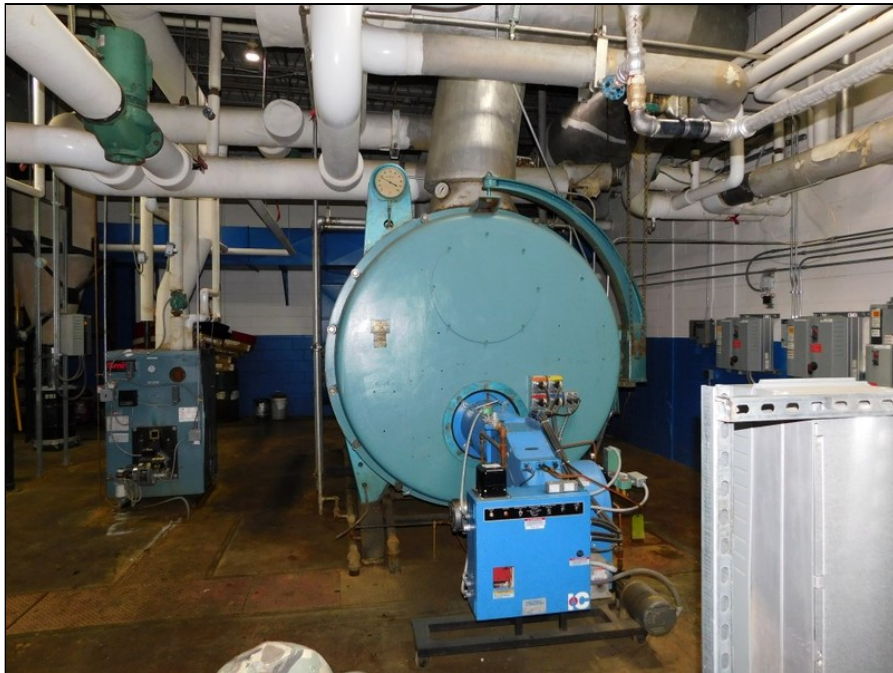
84 - oil fired boiler 1
