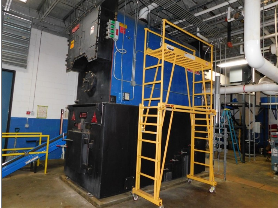
83 - wood chip boiler
