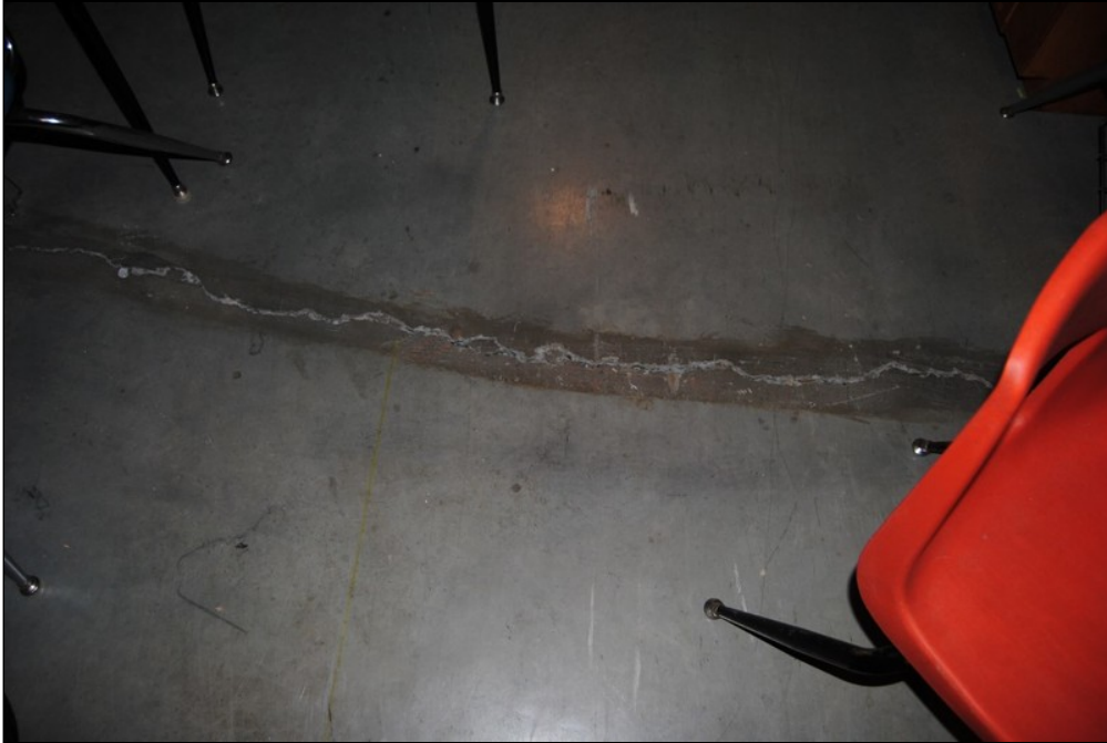
43 - cracked elevator slab
