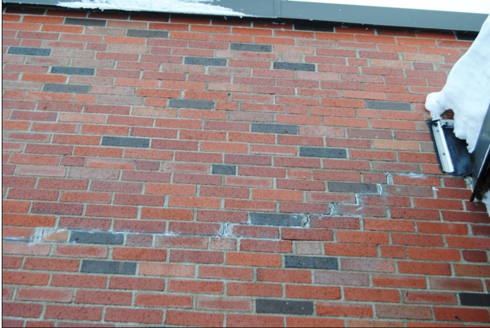
25 - step cracking
