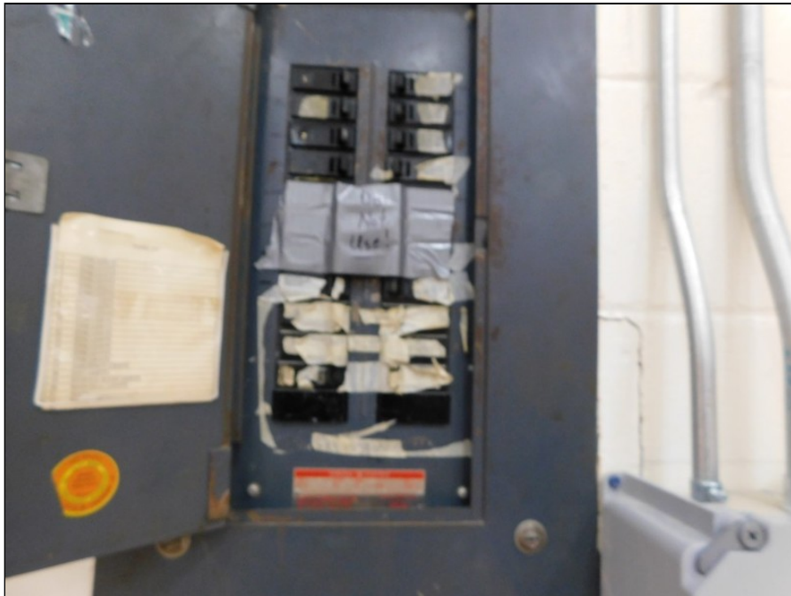
2 - taped over breakers
