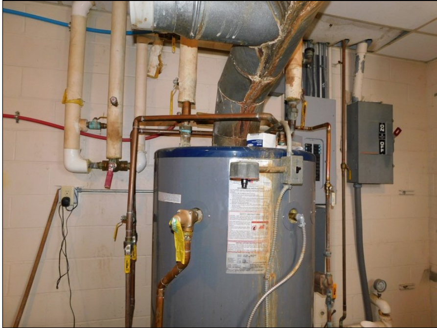
71 - oil fired water heater
