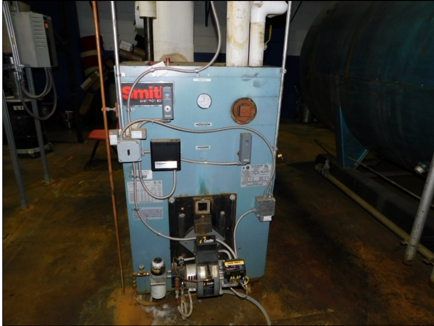
85 - oil fired boiler 2
