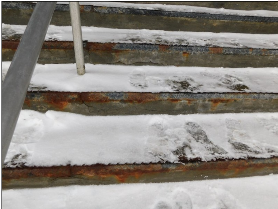
4 - failing entry stais
