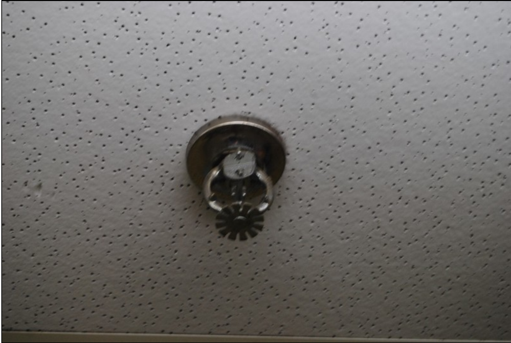
9 - fire sprinkler head
