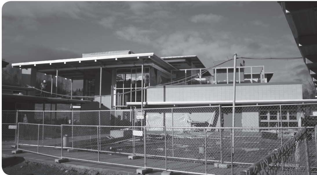
THE 18-CLASSROOM INSTRUCTIONAL WING AT KENMORE JUNIOR HIGH SCHOOL WILL BE COMPLETED BY DECEMBER 2012.
